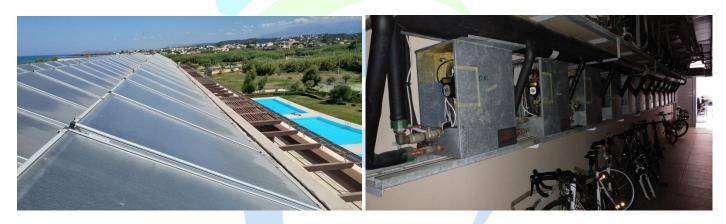
On the right hand side picture you can see 12 heat exchangers, that reheat water via cooling the Freon from the A/C units. Then the reheated water is being sent to the spa pool without the use of any other heat source.
